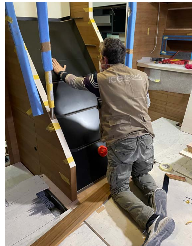
ACCURATE AND CAREFUL ASSEMBLY OF THE SOUNDPROOF STAIRCASE
